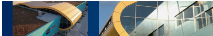
In the spirit of Feng Shui: Rhepanol hg on the shopping centre "Life" in Munich.
